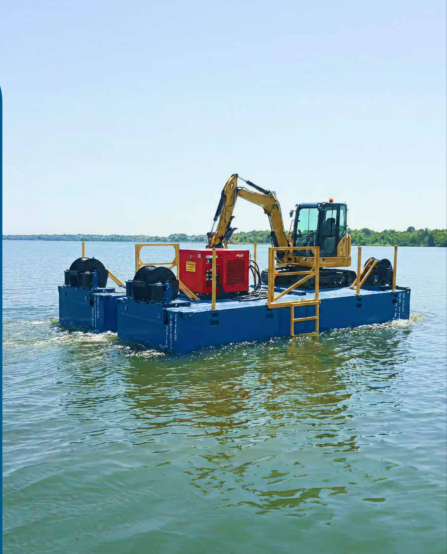
ModBarge creates multimodal floating platforms
