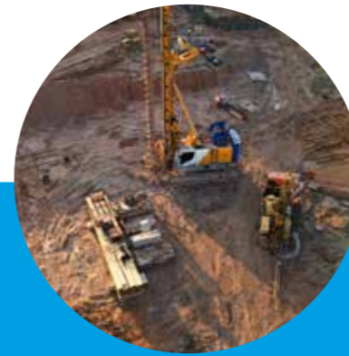
PILE DRIVING GEOTECHNICAL WORK
